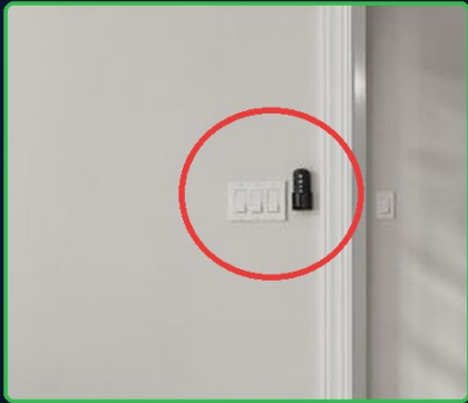
BEFORE switch plate + keypad
